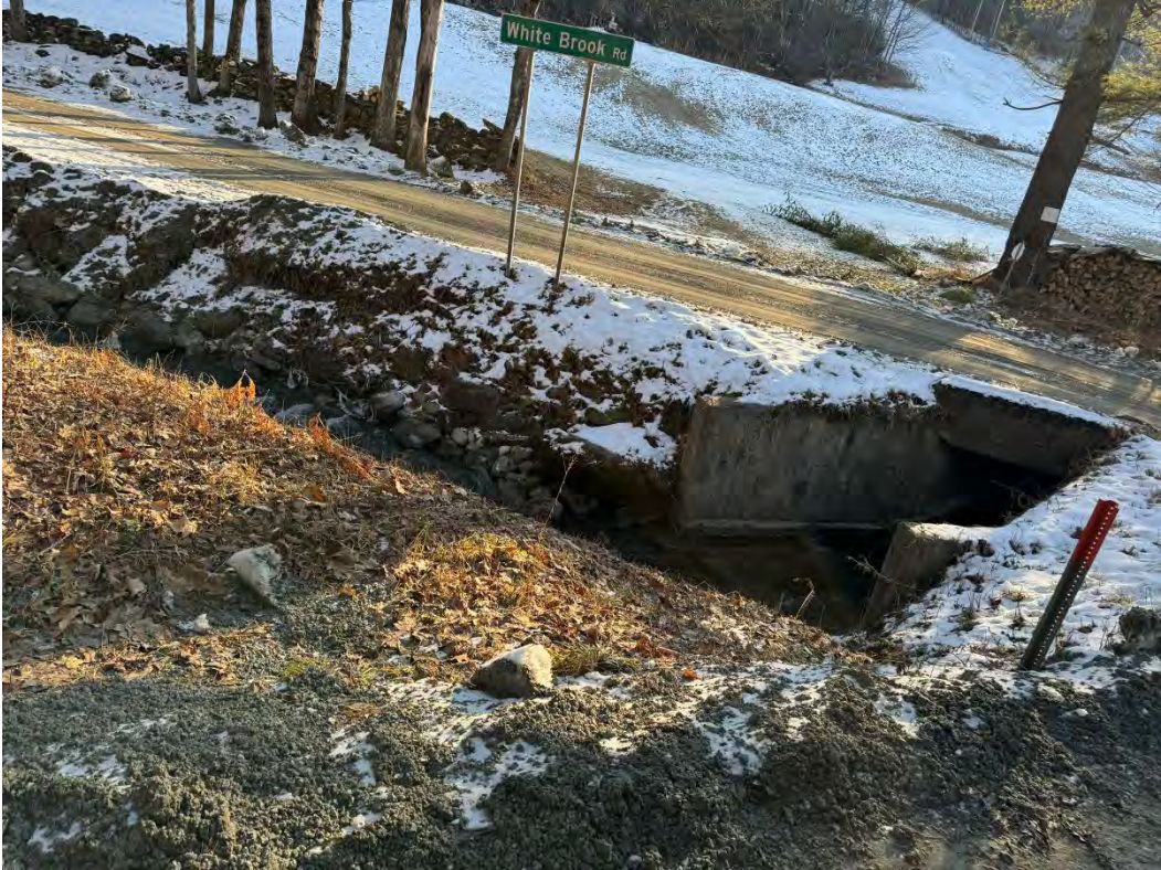
185725 before 2 – replace 15" culvert with 18" feeds into tributary
