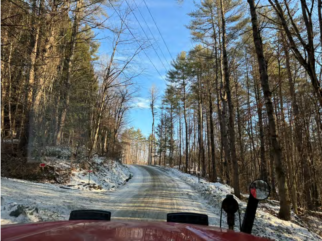
185732 before 1 - heading uphill, install stone line ditch left side above driveway
