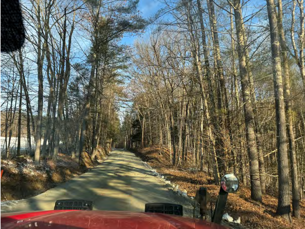
185325 before 1 – heading uphill, install stone line ditch both sides, tree removal
